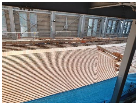
Restoration of the roof of the main hall at Enryakuji temple.
